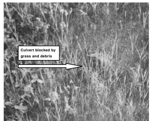
Culverts in a number of locations were observed to lack recent maintenance. Culverts should be marked with painted wood posts to reduce damage from
